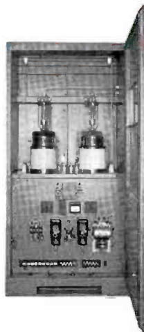
Front view of modulator cabinet. The 21A control system affords complete circuit protection.
